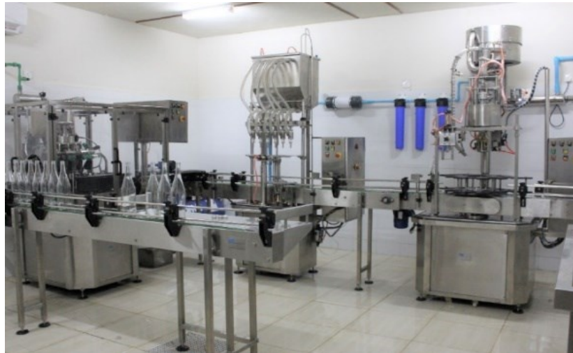
Figure 5 Reverse osmosis system (bottling plant water) [Source: eco-purify.com, 2020]
